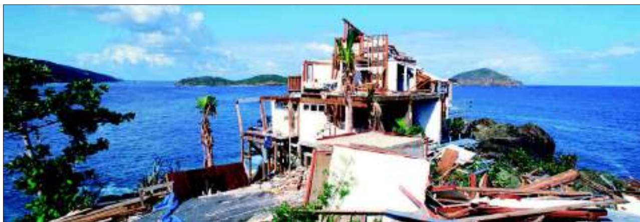
Destruction after hurricane
